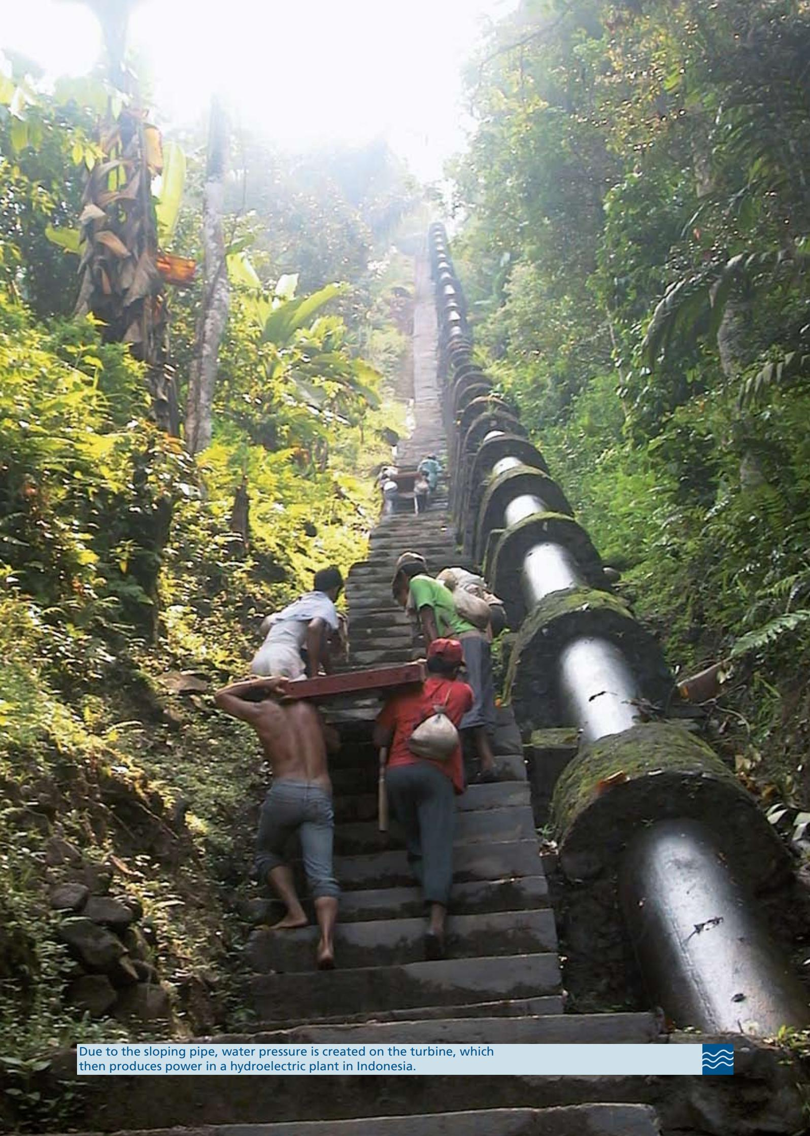
Due to the sloping pipe, water pressure is created on the turbine, which then produces power in a hydroelectric plant in Indonesia.
