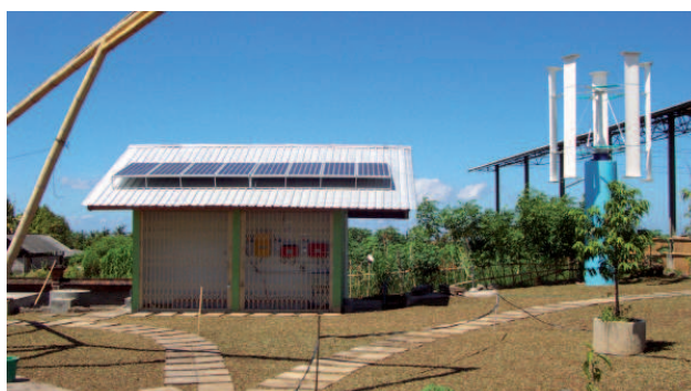
The photovoltaic cells and the wind turbine are part of the Education Park.
