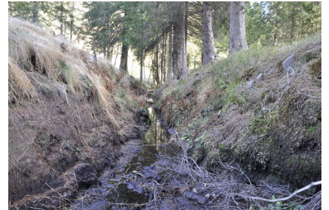
Drainage ditch. This is filled in during rewetting.
