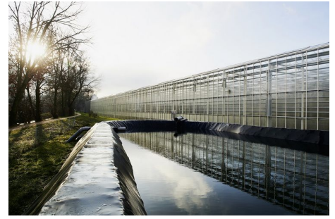
Rainwater basin as storage for 1'800 cubic meters of rainwater for the irrigation of salads. Photo: Forster Gruppe
