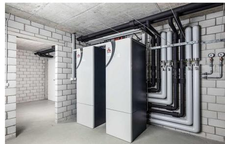
By arranging them in a cascade, heat pump systems can also achieve very high heat outputs for apartment buildings. Copyright: CTA AG
