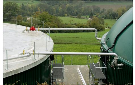
A double-membrane roof on the fermentation tank and a covered final repository for fermentation residue ensure that no methane escapes into the atmosphere (Foto: Klimastiftung Schweiz).
