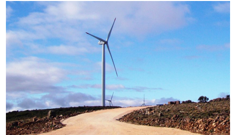
The six wind turbines deliver clean power from renewable energy for more than 100'000 households
