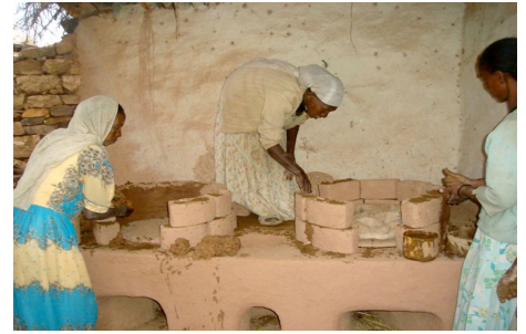
Working together, the women erect the upper part of the mogogo oven with prefabricated tiles.
