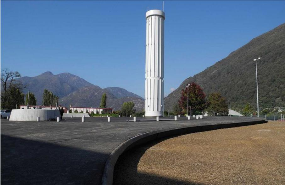
The chimney above the underground wood chip heating plant. The heating plant provides the school building (red building in background) and other buildings with heat from renewable energy.
