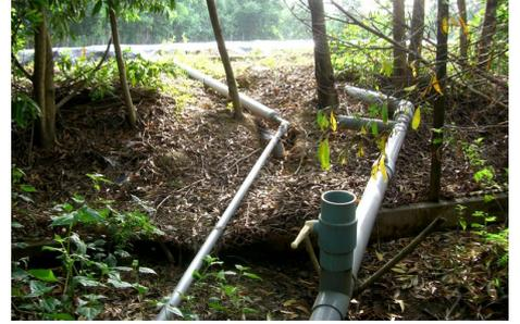
The captured biogas (methane) is transferred through pipes to the boilers where it is burnt to generate electricity.
