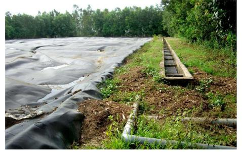
A membrane captures the climate-damaging methane gas.
