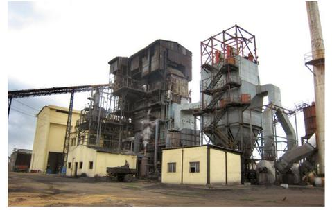
In the power plant, the biomass is used as efficient fuel for energy production which is fed into the regional power supply system.
