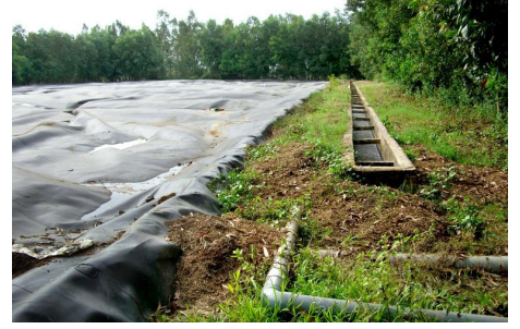
A membrane captures the climate-damaging methane gas.
