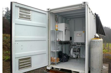
View into the control container. A data logging system provides continuous measurement data.
