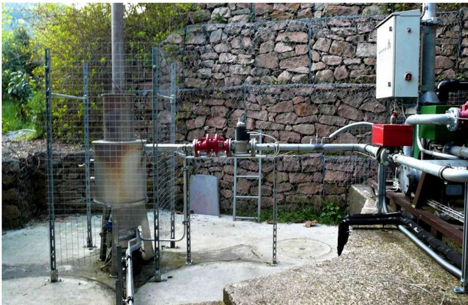
Workers installing the low-gas torch in Croglio, which due to modification, will be able to keep burning off rubbish tip gases for decades into the future.
